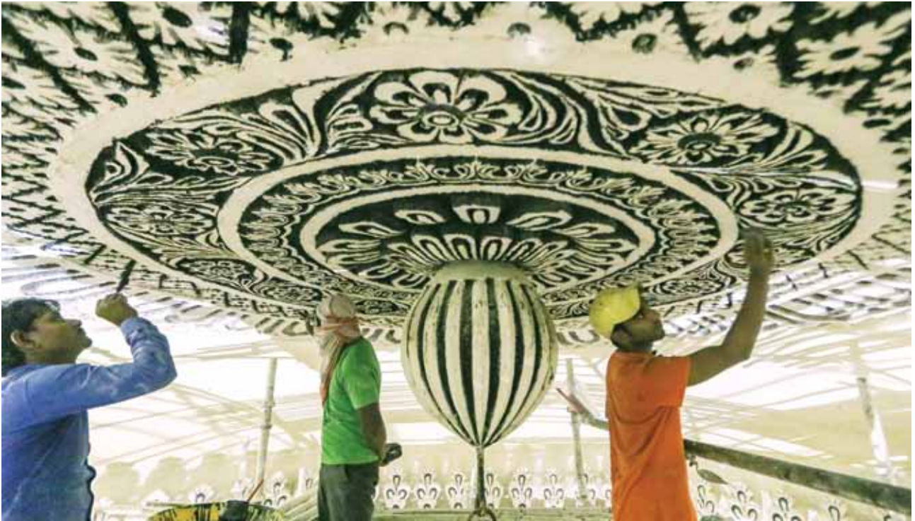
Restoration of an ornamental ceiling medallion in the mausoleum of Abdullah Qutb Shah by traditional lime craftsmen. Image courtesy: Aga Khan Trust for Culture
