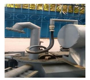
Tata Power Delhi Distribution Limited (Tata Power-DDL), a leading power utility supplying electricity to over 2 million customers in North Delhi, has been granted the patent for its unique Self-regenerating Transformer Breather for a term of 20 years. The 'Self-Regenerating Breather' is a device that protects a transformer from moisture ingress and thus, increases the longevity of electric transformers.
